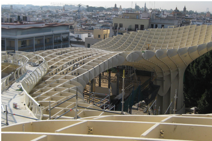
Figure 4. Machined Kerto LVL in Metropol Parasol Sevilla, Spain
