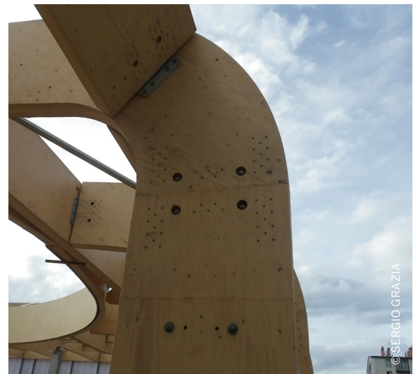
Figure 1. Curved Kerto LVL in Clamart Sports Complex, France
