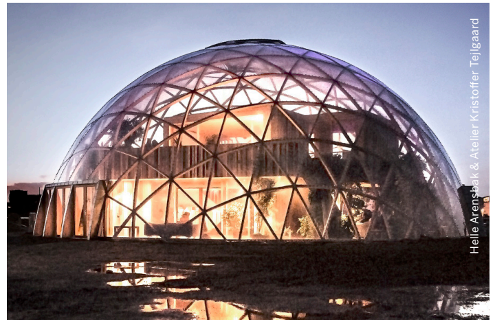
Figure 5. Bent Kerto LVL in Dome of Visions 3.0, Denmark
